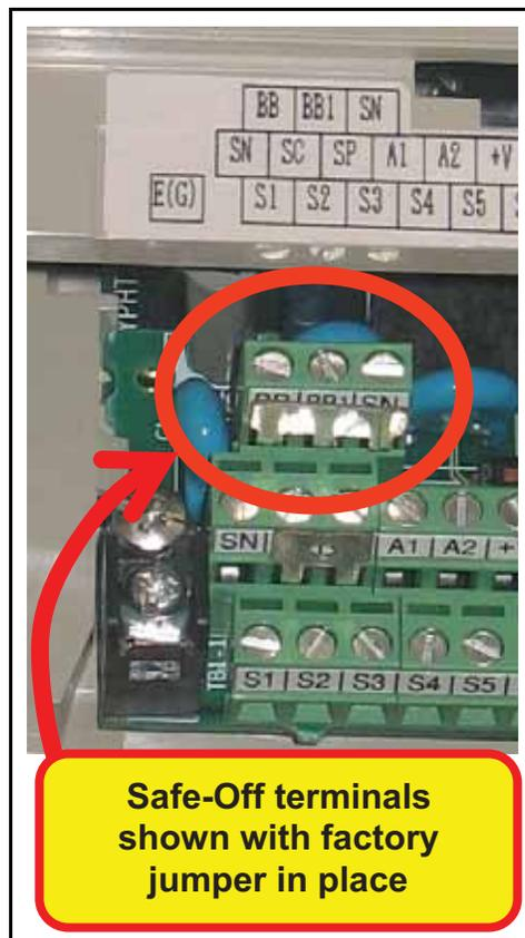
The time from opening either Safe-Off input until the drive output is switched off is less than 10 milliseconds.
